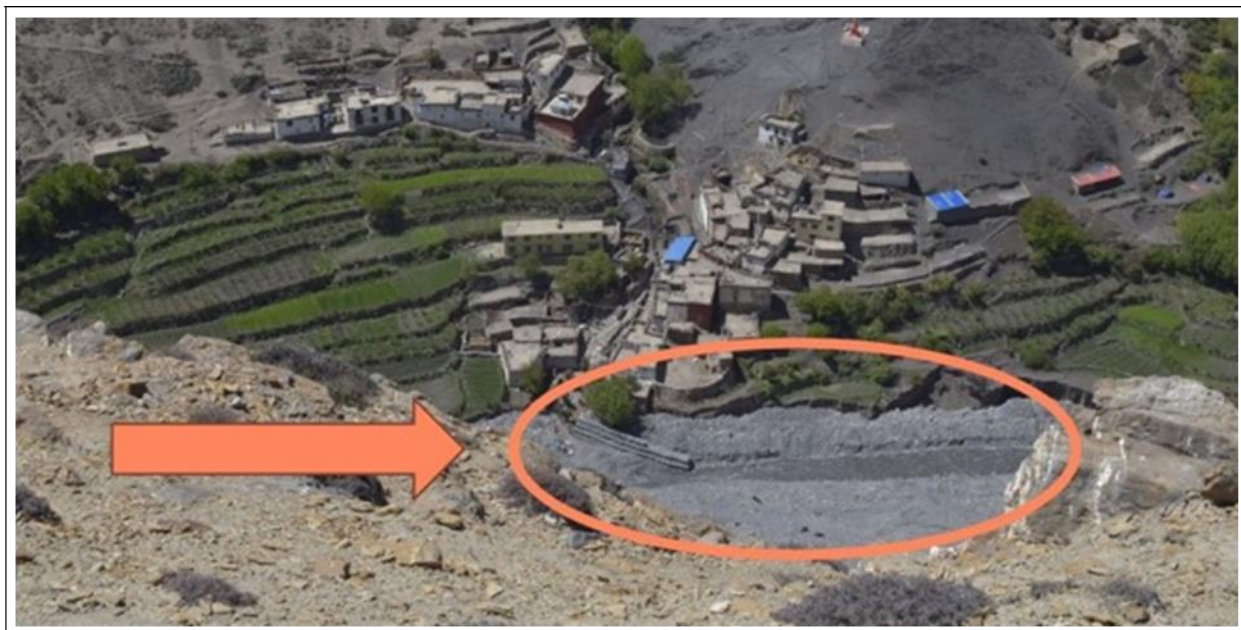
Figure 7: Trench and Gabion Boxes Guarding the Main Village in 2021
